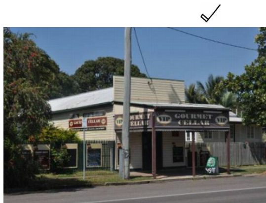
Figure SC6.2.4.2 Existing acceptable example of a non-residential use in an acceptable non-residential building (no setback to street boundary and awning over footpath)
